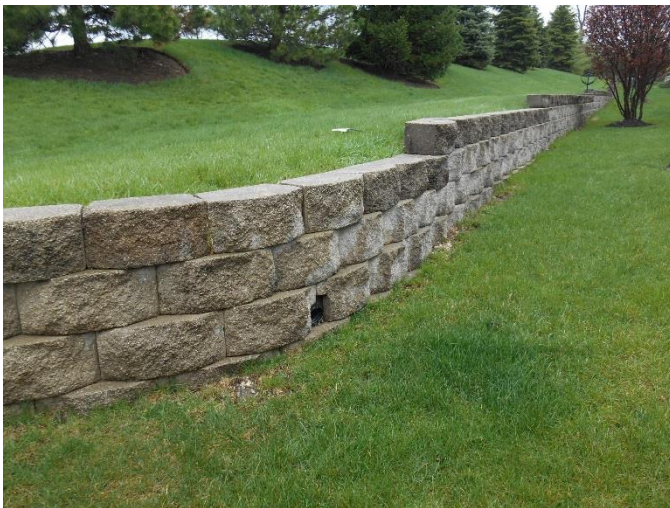
Typical retaining wall.
