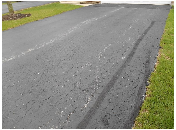
Typical asphalt driveway.
