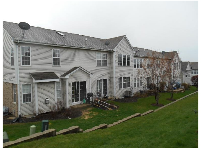
Rear elevation with no balconies or decks.
