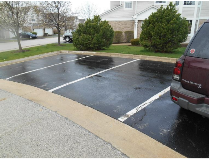
Typical asphalt parking area.
