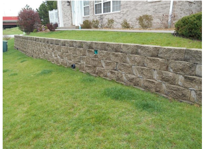
Typical retaining wall.
