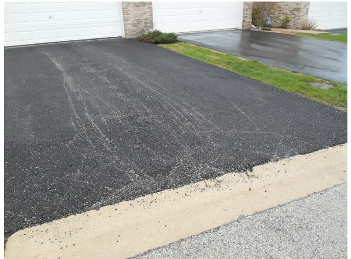
Recently replaced driveway.
