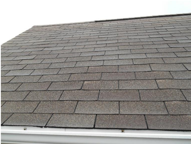
Overview of roof shingles.
