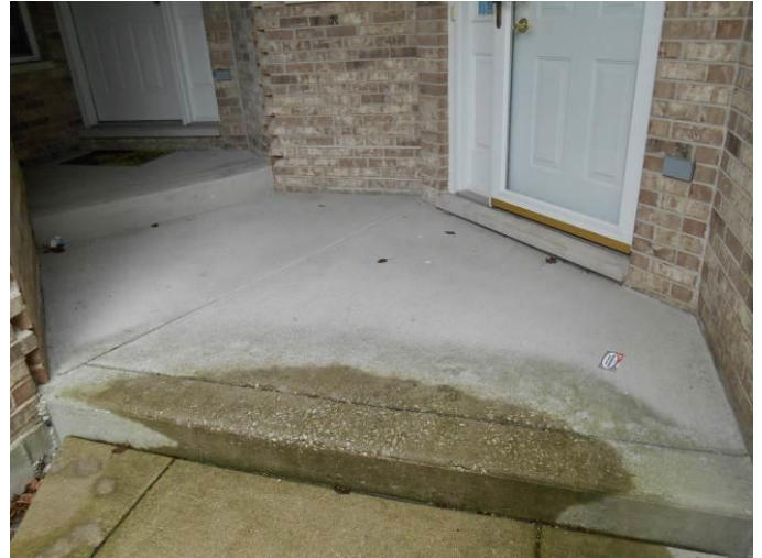
Interior unit entrance stoop.
