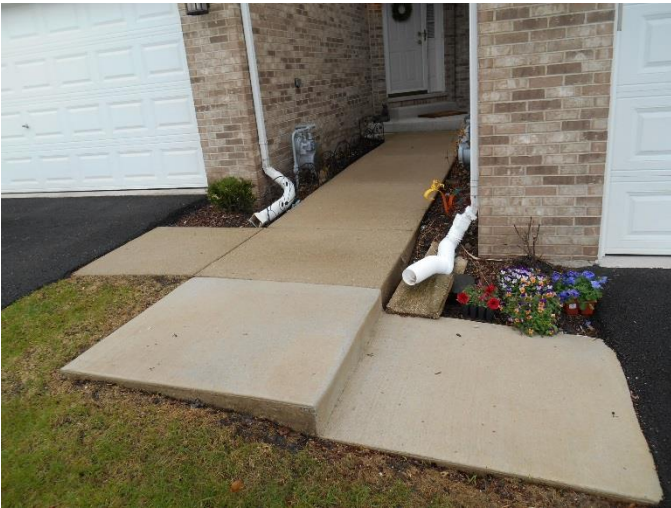
Recently repaired walkway.
