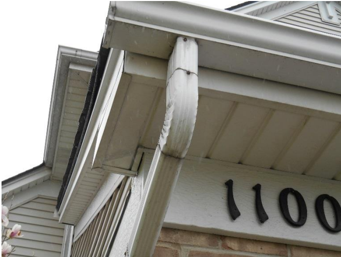
Gutters, downspouts, soffit, and fascia.
