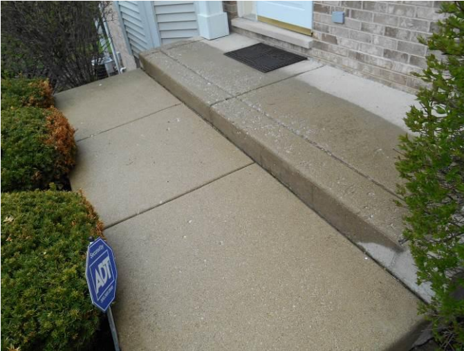
End unit entrance stoop.
