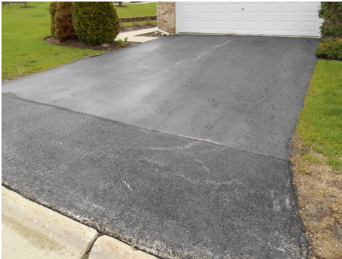
Recent driveway repair.
