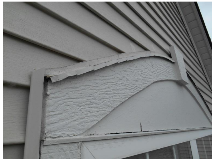
Siding and wood trim detail.
