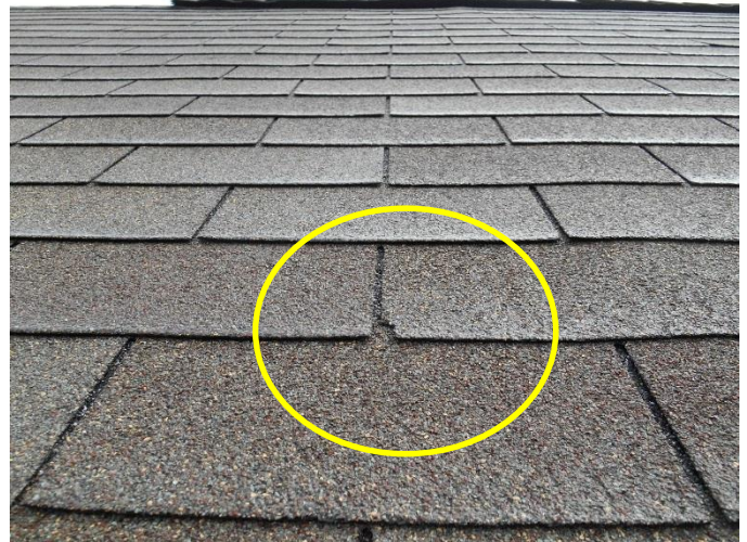
Deteriorating shingles.
