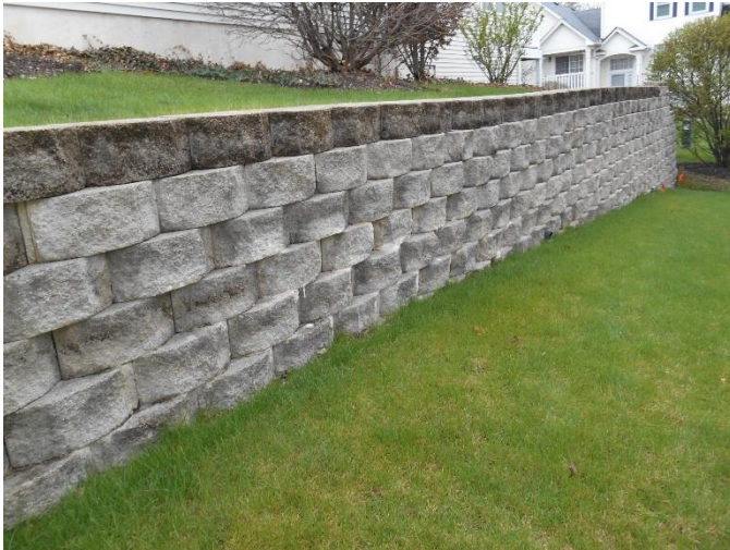
Typical retaining wall.
