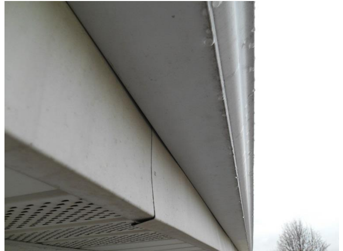
Gutters, soffit, and fascia.
