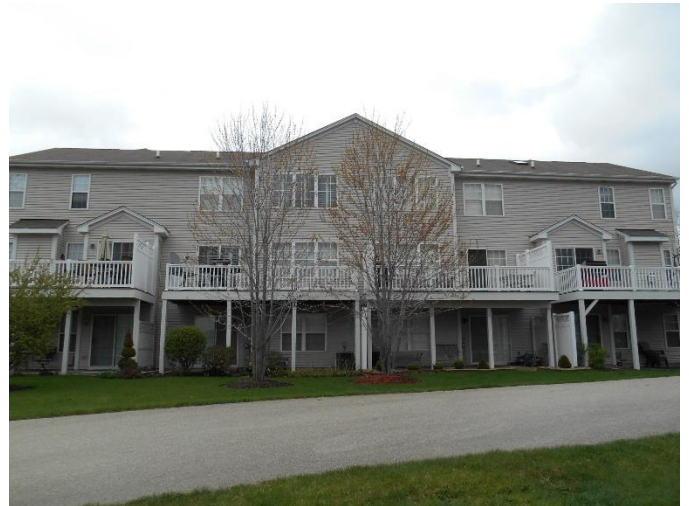
Rear elevation with balconies.
