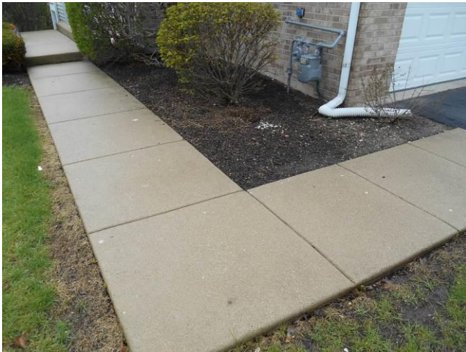
End unit walkway.
