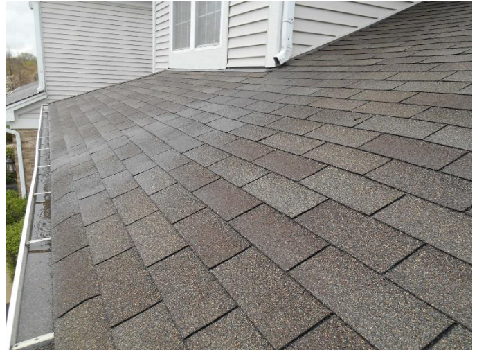
Overview of roof shingles.
