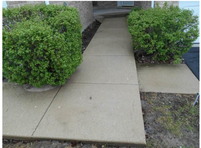
Interior unit walkway.
