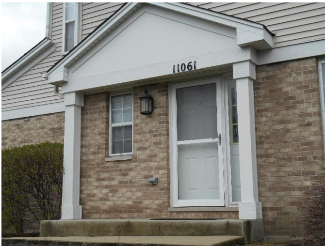
End unit entrance brick, siding, and wood trim.
