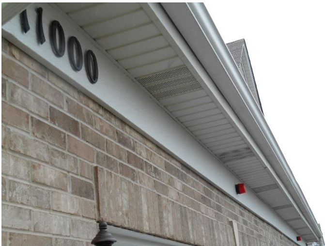
Gutters, soffit, fascia, and wood trim.
